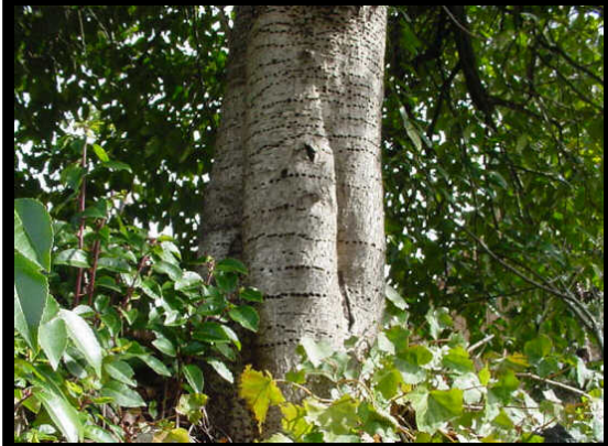
~ Caption: Sapsucker damage on birch ~ Photo by: C.R. Foss
